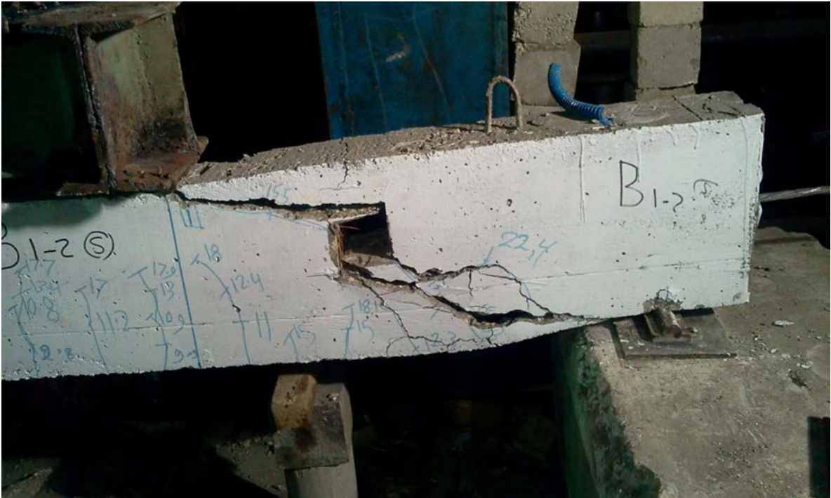
Photo (6) Failure of the tested beam {B1-2 (S)}.
