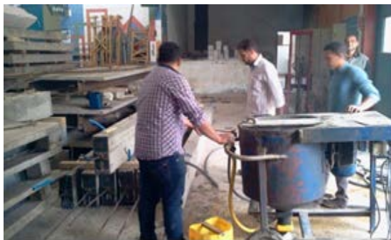
Photo (2): Injection the grouting
