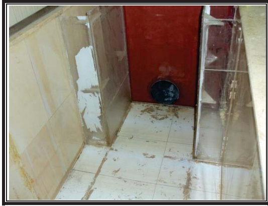
Photo (3) The Outlet of the Syphon.
