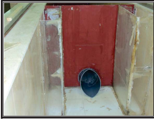
Photo (2) The Inlet of the Syphon.
