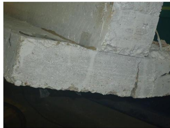
Photo (4): Failure Shape of Rectangular Strip Footing.
