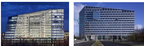
North - South façade of The Edge Building
