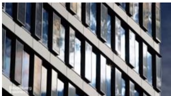
Fig 14. The solar panels act as Louvers on the south facade of The Edge building.
