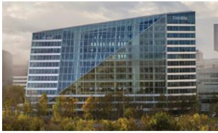
Fig 1. The usage of large glass openings on the north facade of the building and Slope in the surface of the atrium
