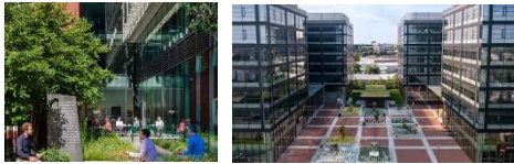
Courtyard of 2100L Street NW and J8 Office Park
