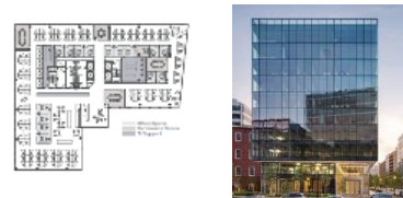
2100L Street NW Building - Southeast facade
