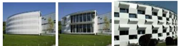
Fig 4. The Kiefer Technic administrative building in Australia shown with all louvres closed and open.
