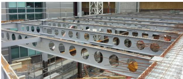
Figure 2 Castellated beams application
