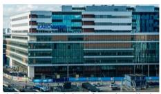
Fig. 4: Facades consisting of curtain walls that can be easily changed and replaced whenever required. Karolinska Hospital, Stockholm, Sweden.
