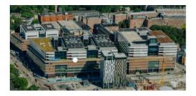
Fig. 1: The compact shape of a new Karolinska Solna Hospital with the provision of internal courtyards due to the importance of lighting and natural ventilation for patients and users.
