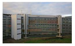
Fig. 5: New Martini Hospital in Groningen. Central stations such as steam boilers, refrigeration stations, compressed air, etc. are located on the rear facade which extends to the roof through insulated pipes. The fixtures are placed in a central column for each building block, which consists of 80% public spaces and 20% specific spatial destinations, and the insulated pipes outside help to maintain the best arrangement of the future space [8].
