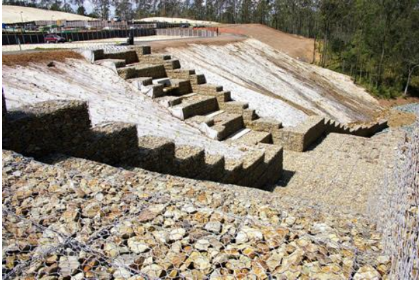
Figure 1 gabion structure. Brisbane, Queensland, Australia.
