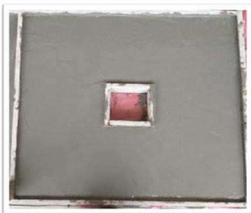
Fig.4. Finish of casting process at the concrete slab with central opening
