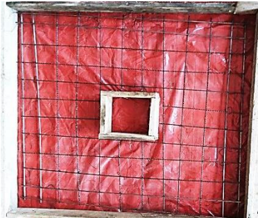
Fig.3. Reinforcement in the wooden form
