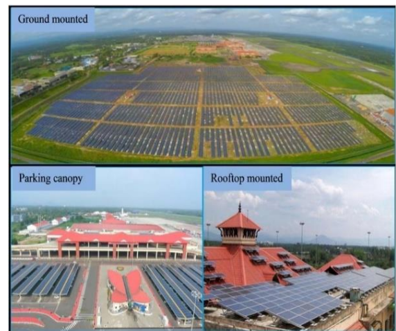
Fig. 1: PV Plant on International Airport in India [9]
